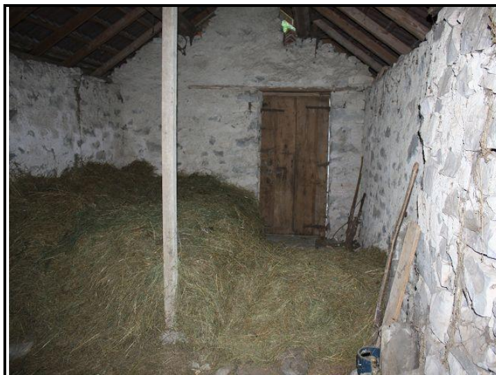
Locale sopra / Dachraum
