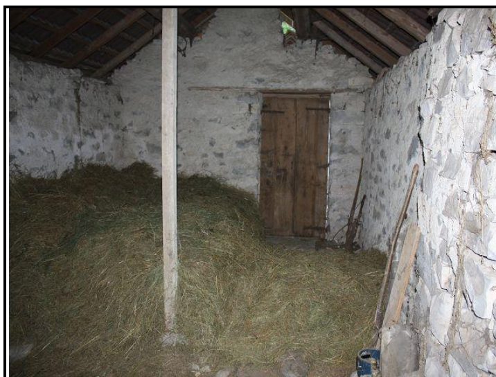
Locale sopra / Dachraum
