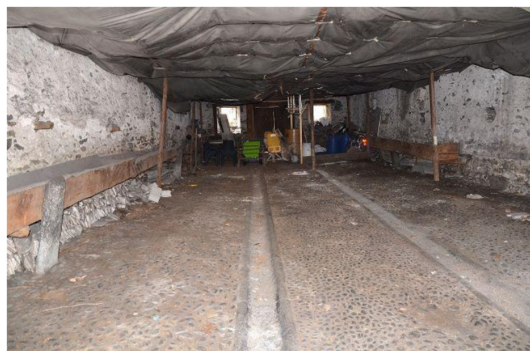
Innenraum Erdgeschoss / piano terra
