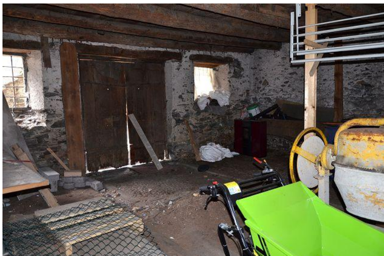
Innenraum Erdgeschoss / piano terra
