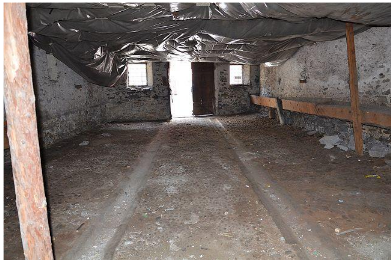
Innenraum Erdgeschoss / piano terra
